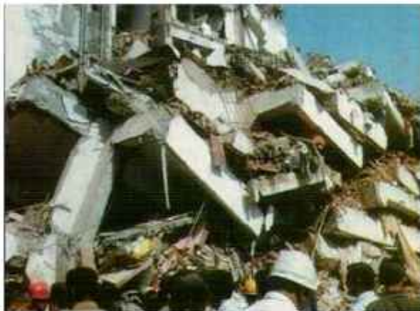
Damage due to earthquake
